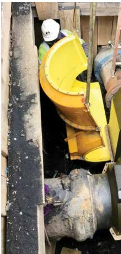
*A custom-made mold is lowered into the excavation before being installed onto the leaking fitting*
