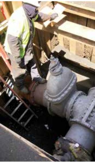
After descaling and sandblasting, the fitting is ready for primer
