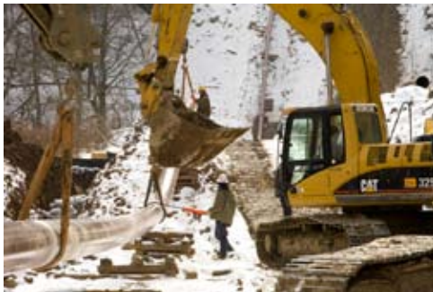
Crews carefully lower the pipeline into the trench
