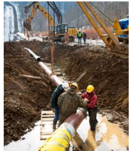
Crew members perform field tie-ins
